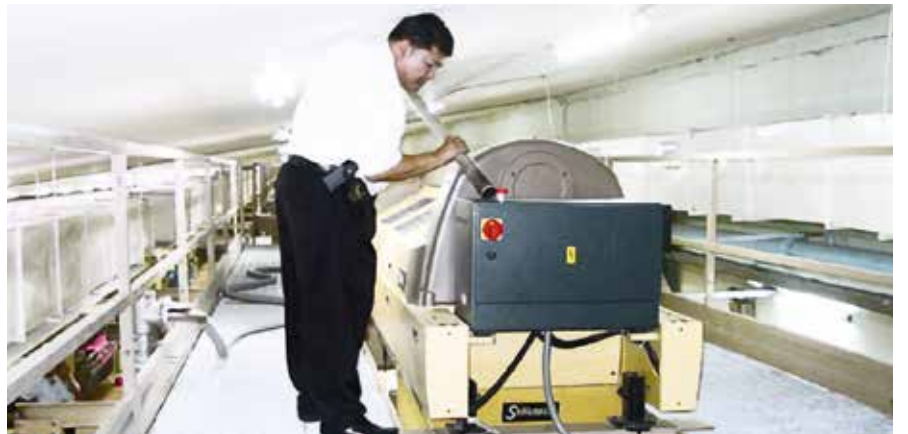
Manual Cleaning at Gantry Level
