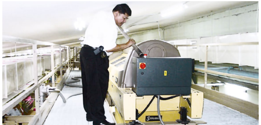
Manual Cleaning at Gantry Level
