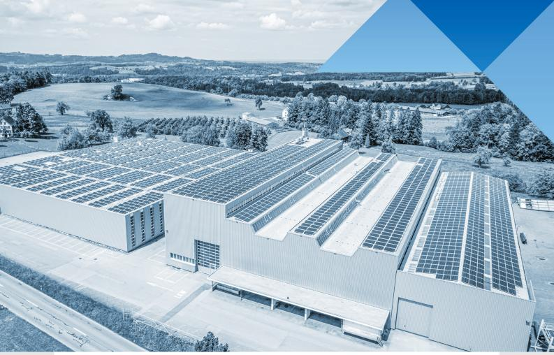
Photovoltaic system: 1'924 modules = 3'146 m" | plant performance: DC 442.24 kWp | AC 372.80 kVA
