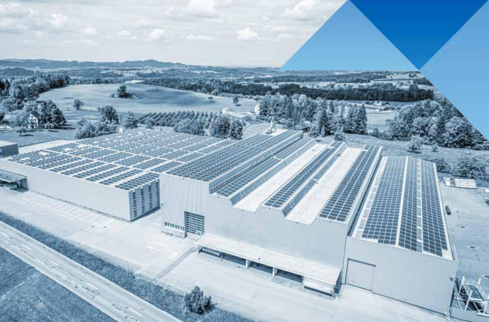
Photovoltaic system: 1'924 modules = 3'146 m<sup>2</sup> | plant performance: DC 442.24 kWp | AC 372.80 kVA
